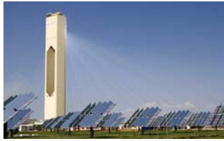
Seville's PS10 solar power tower plant generates 11 megawatts from 624 heliostats. Nearby PS20, currently under construction, will be twice as powerful
